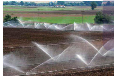
Commercial/Agricultural irrigation system
